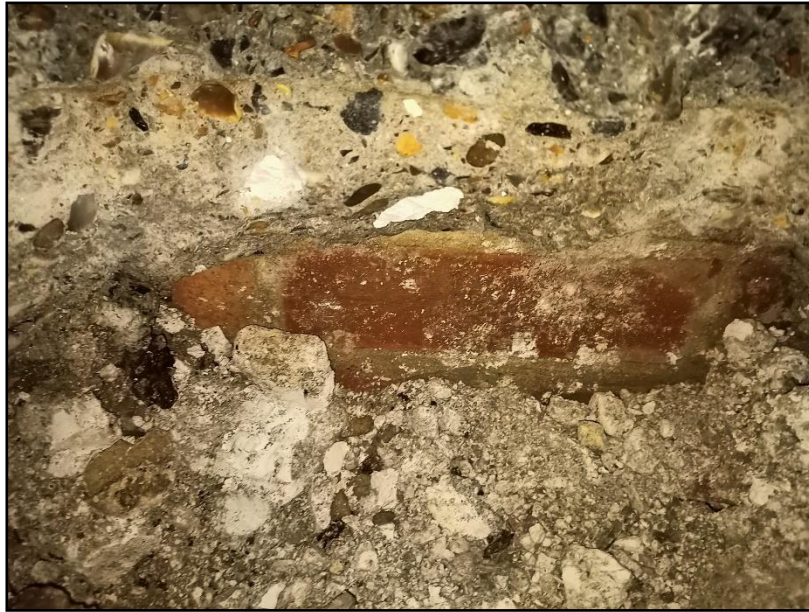
(Fig 18 – Looking south at Section 5)
