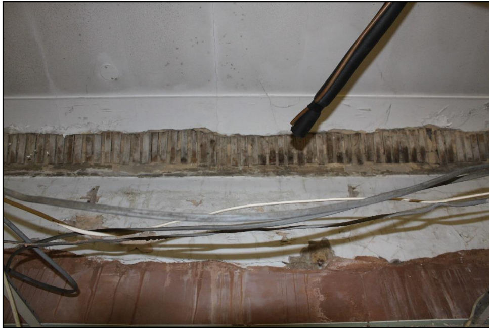
(Fig 22 – Lathe plasterwork exposed in-ceiling coving)
