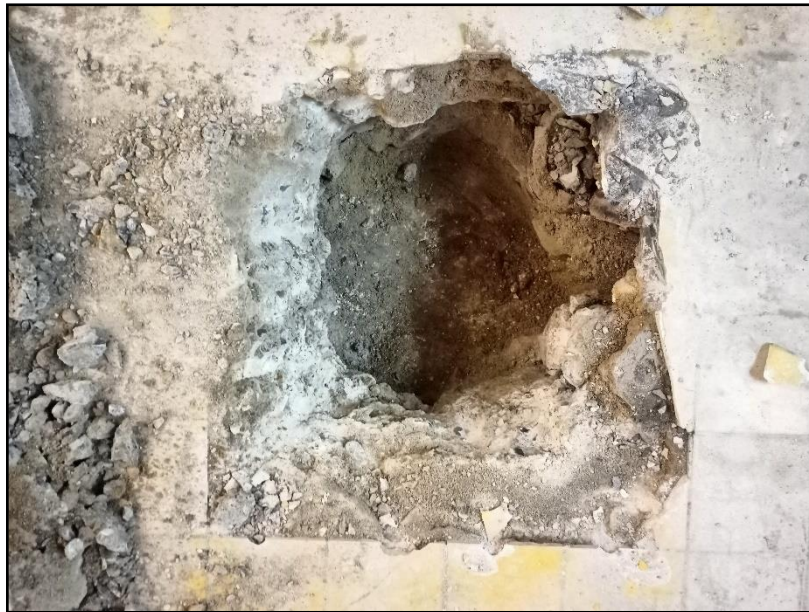
(Fig 19 – Looking overhead test pit 5 / borehole 2)
