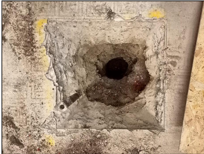
(Fig 20 – Looking overhead borehole 1)
