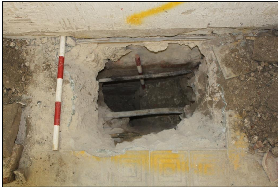
(Fig 13 – Looking south at Section 3)
