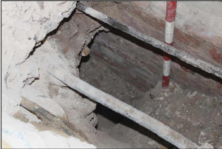
(Fig 14 – Oblique view of Section 3 showing internal-faced brickwork of 1008 to a depth of c.1.0m and backfill 1004 abutting the likely cellar wall)
